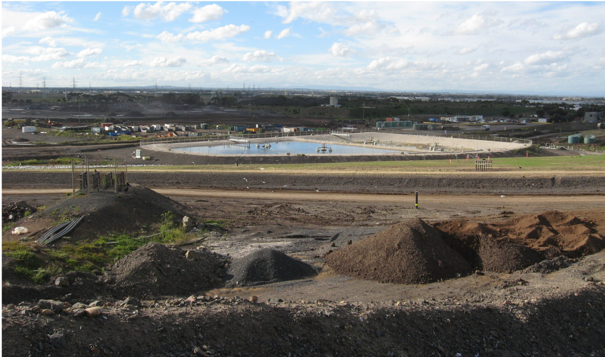
Figure 4: View towards northeast across Stage 2 (existing landfill) showing the leachate pond (centre of photo)
